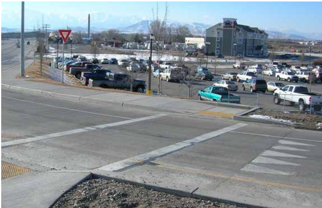
Exhibit 1-9. Pedestrian crossing at the right-turn lane of the exit located at Pioneer Crossing and I-15 DDI (American Fork, UT). (6)
