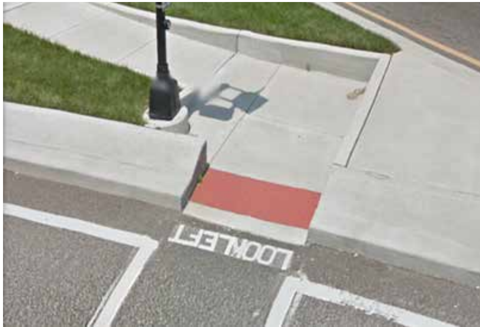
Exhibit 8-27. Engraved pedestrian pavement marking – “Look Left.” (26)
