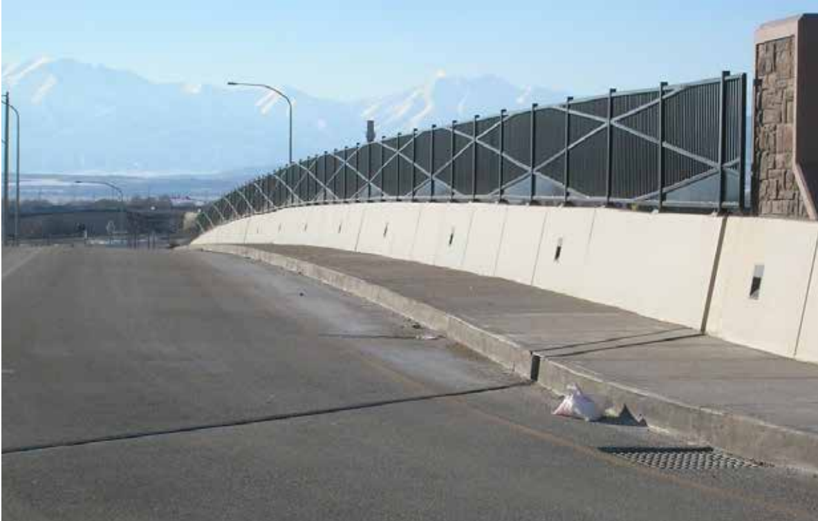
Exhibit 1-10. Sidewalk and recessed lighting located on the bridge at the Pioneer Crossing and I-15 DDI (American Fork, UT). (6)
