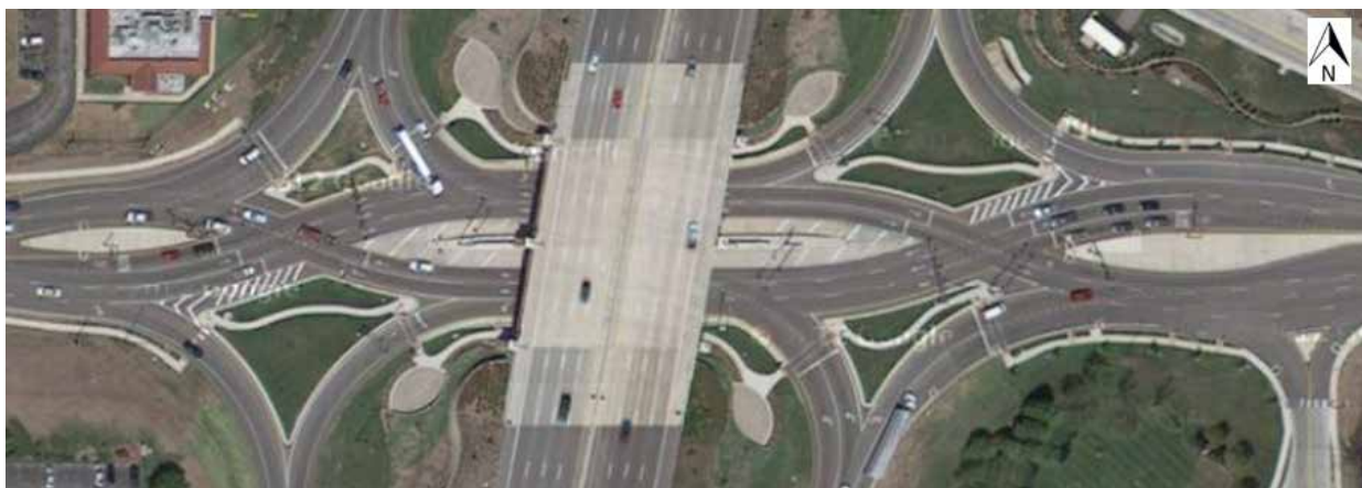
Exhibit 7-12. Shifted alignment south of centerline (red) with no reverse curves between crossovers (Pioneer Crossing, American Fork, UT) (26)
