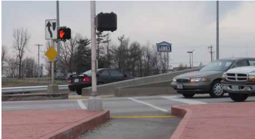
Exhibit 8-13. Pedestrian signal and push-button on outside of crossover (pedestrian facilities in center). (14)
