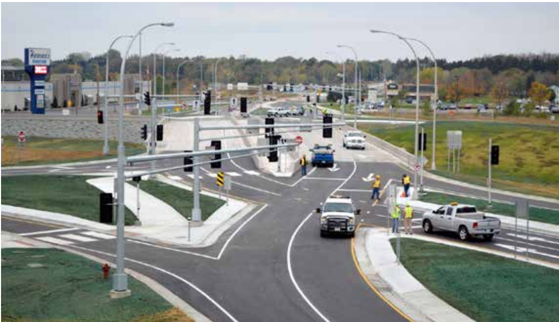
Exhibit 1-5. First constructed DDI in Minnesota at Highway 15. (3)
