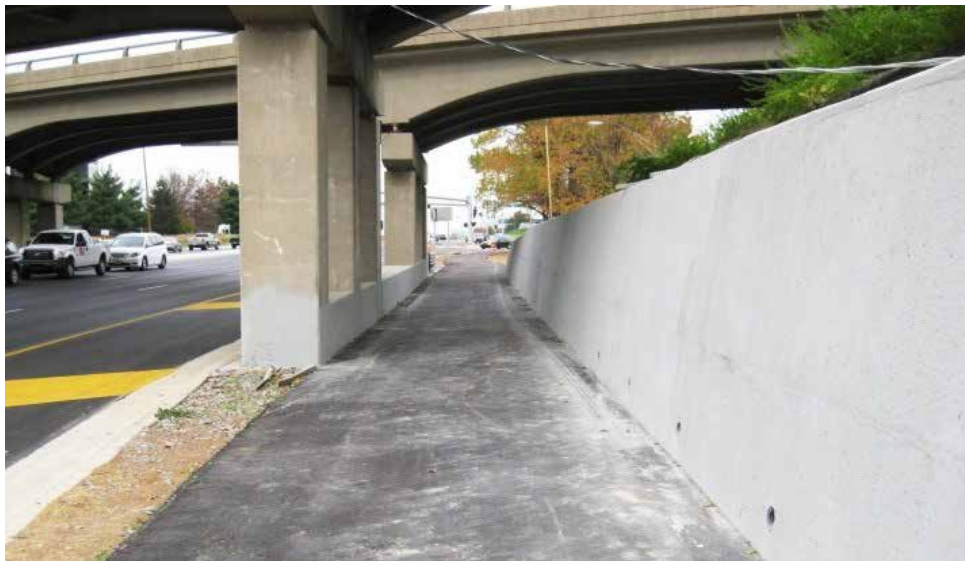
Exhibit 3-4. Shared-use path on outside at Harrodsburg Road (Lexington, KY). (14)
