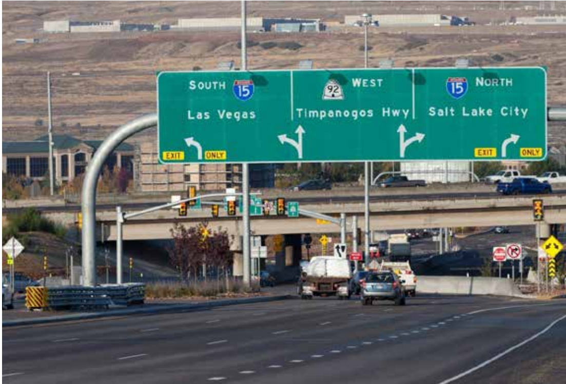
Exhibit 1-8. Overhead signing at the DDI located at SR 92 and I-15 (Utah County, UT). (5)
