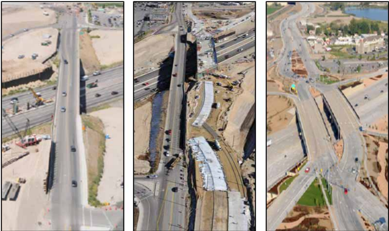
Exhibit 9-3. Construction staging using pre-cast construction methods. (48)
