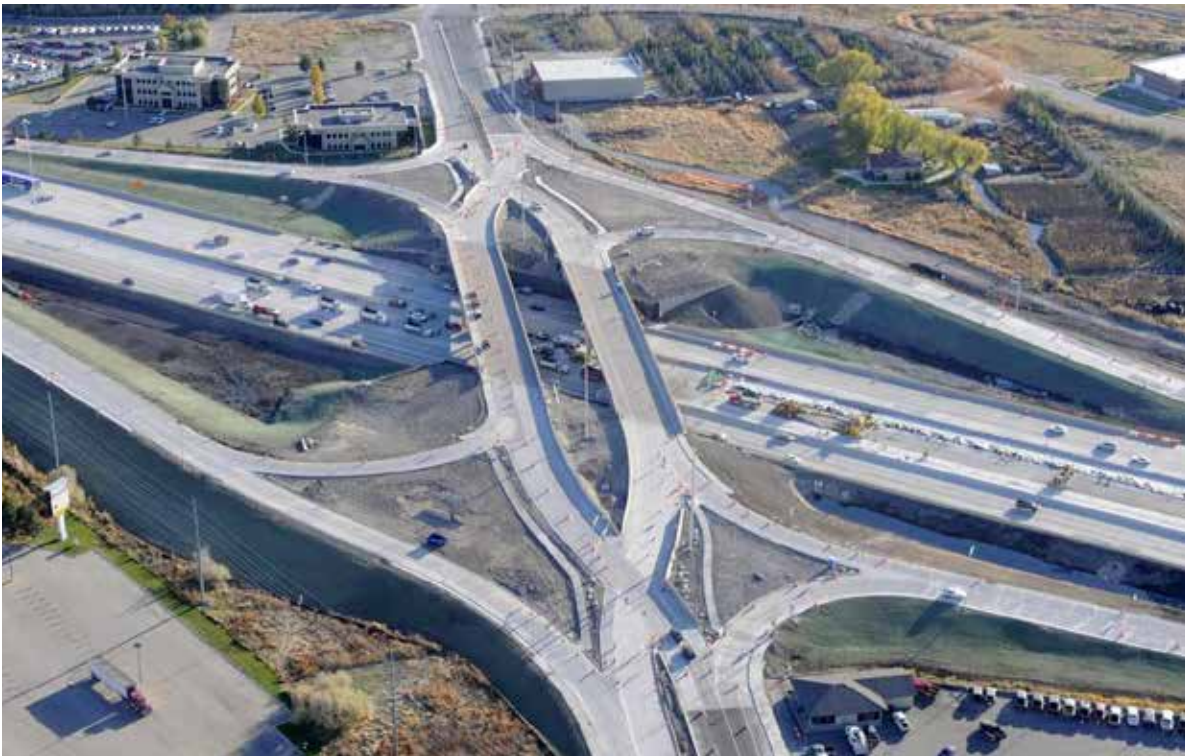
Exhibit 1-11. DDI (overpass) at 500 East American Fork (American Fork, UT). (1)
