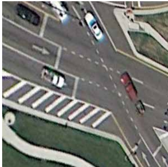
Exhibit 4-9. Pavement marking used to channel vehicles through crossovers. (26)
