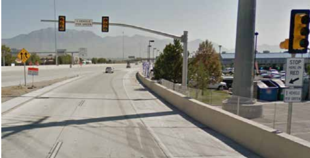
Exhibit 5-10. Ramp meter with added lane for queue storage at a DDI. (6)
