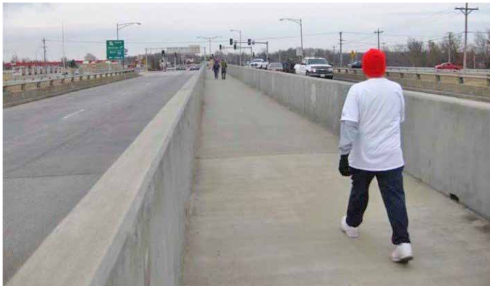
Exhibit 3-2. Center walkway at MO 13 (Springfield, MO). (14)
