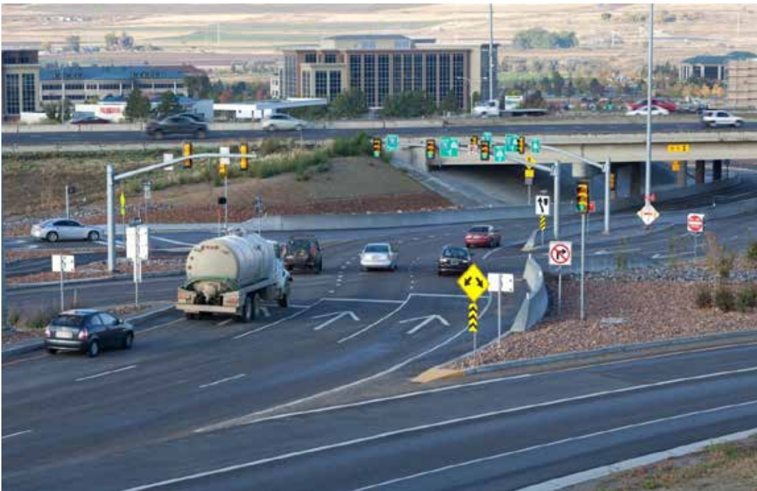
Exhibit 1-7. Crossover location at the DDI located at SR 92 and I-15 (Utah County, UT). (5)
