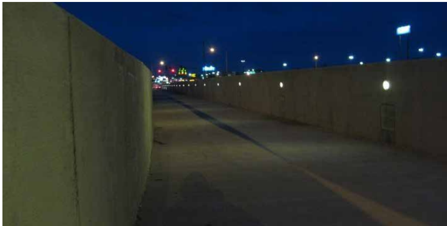
Exhibit 8-31. Recessed lighting in DDI center walkway. (14)
