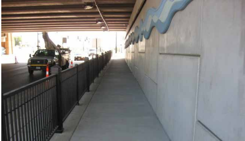
Exhibit 3-3. Outside walkway at Dorsett Road (Maryland Heights, MO). (14)
