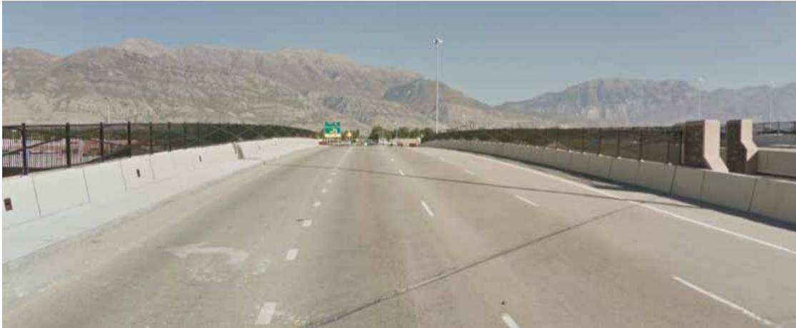
Exhibit 8-22. Use of short skip lines to delineate an exclusive left-turn lane onto a limited access facility. (26)
