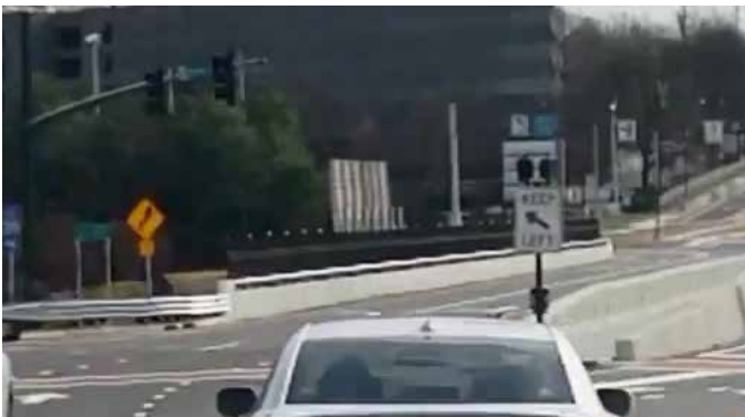
C) Center Walkway, Single Structure Ashford Dunwoody Road - Dunwoody, GA
