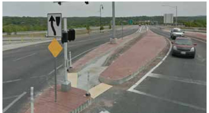
D) Center Walkway, Single Structure MO 248 - Branson, MO
