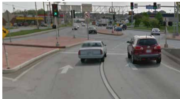
Exhibit 7-15. Barriers and traffic islands to discourage wrong-way movements. (26)
