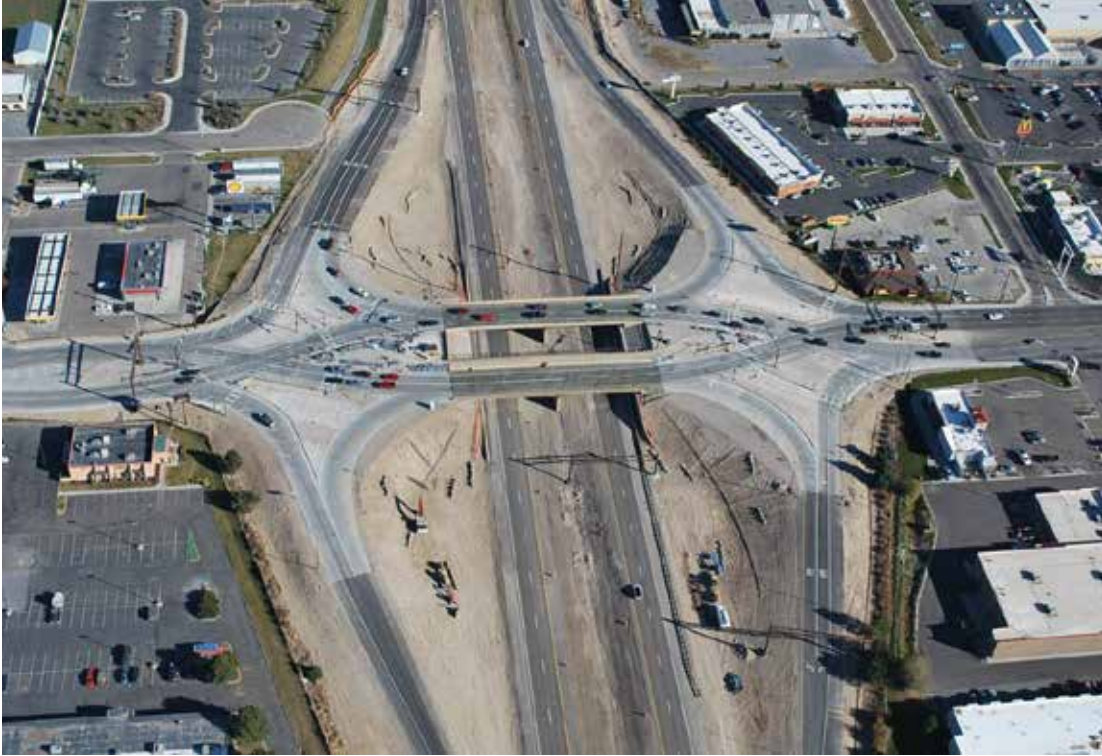
Exhibit 1-6. First constructed DDI in Idaho at I-86 and US-91/Yellowstone Highway (Pocatello-Chubbuck). (4)
