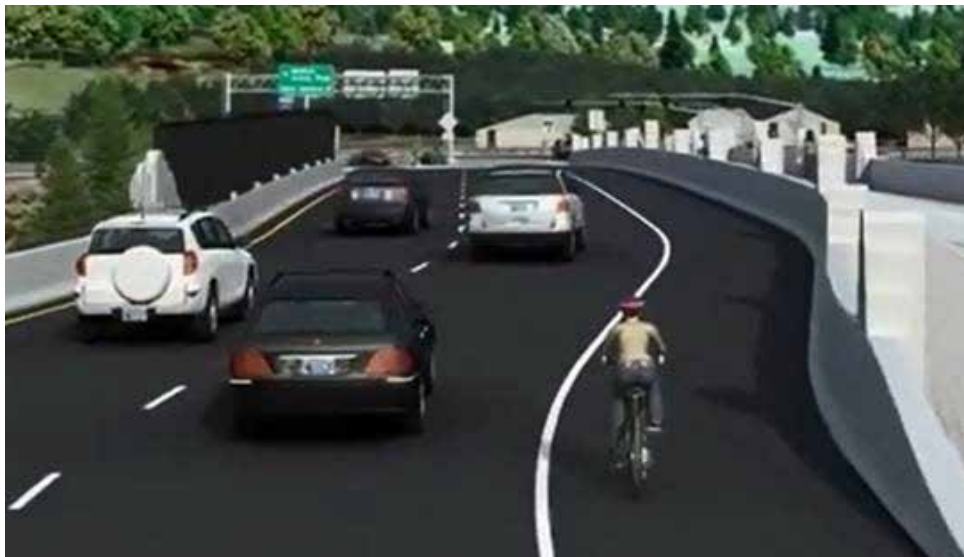
Exhibit 3-22. Bicycle lane maintained through DDI between crossovers. (20)
